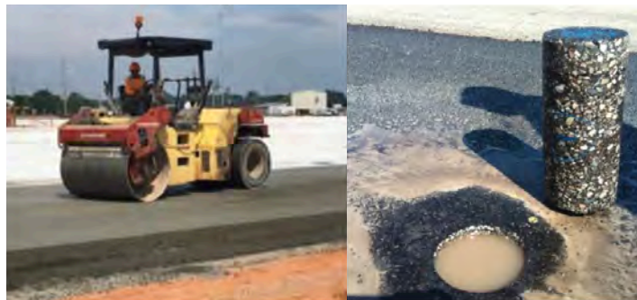
(Left) Pavement design and construction; (Right) Field core extraction for evaluation.
